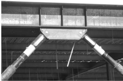
Figure 1. Steel moment frame with dampers
